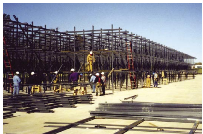
EXTREN® does not rot or corrode, making it the ideal material for cooling tower construction.
