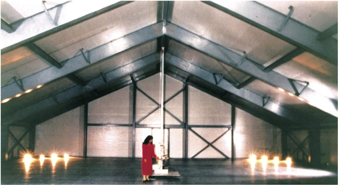
24" (610mm) EXTREN® fiberglass I-beams span 62' (18.9m) wide rigid gables that support the siding and roof of an all-fiberglass building used for computer testing.
