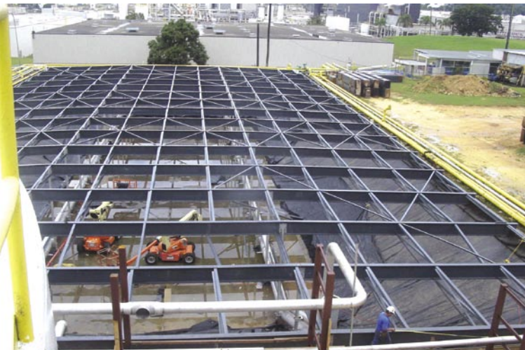
An odor control cover was constructed using EXTREN® structural shapes for a waste water treatment facility in Puerto Rico.
